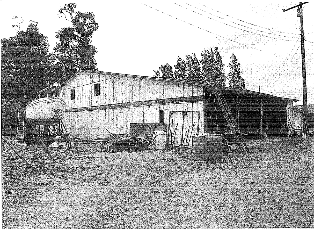
Figure 23 Barn/Living Quarters, south and east elevations (looking northwest)
