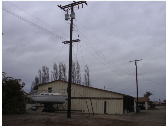
Photograph 2. View of the two pole mounted transformers, barn and attached residence on the eastern portion of the subject property, facing northwest.
