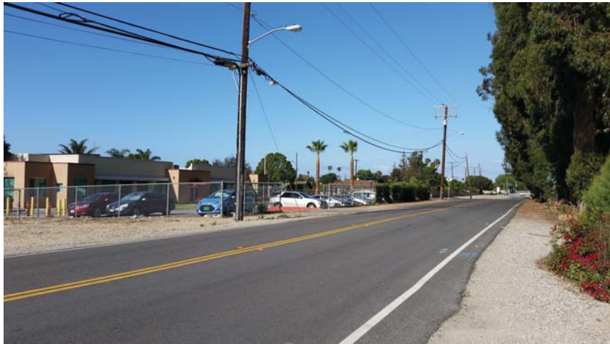
Photo 3: View looking west from project site along Etting Road.
