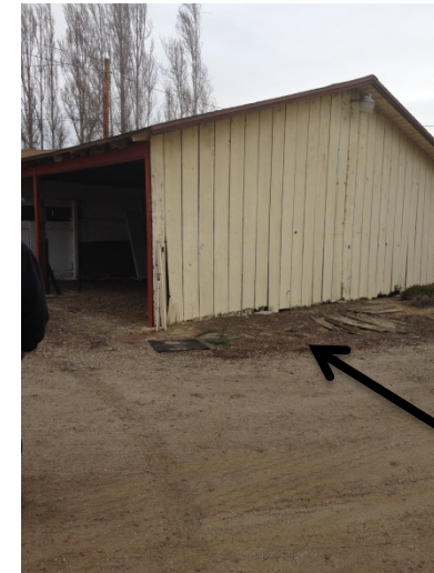
Photograph 12. View of the location where the former underground storage tank was located, facing northwest.
