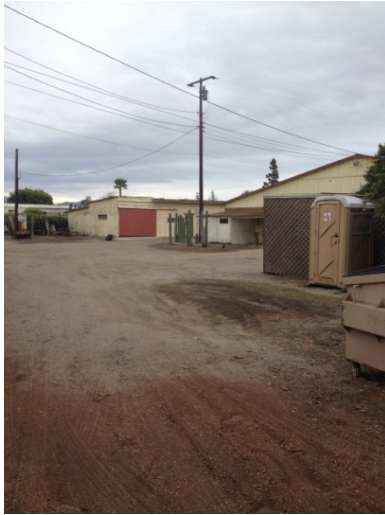
Photograph 7. View of the barn and storage /workshop structure located on the eastern portion of the subject property, facing southeast.
