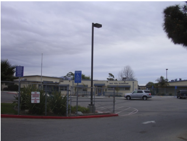
Photograph 16. View of Mar Vista Elementary (2382 Etting Rd.), facing southeast.
