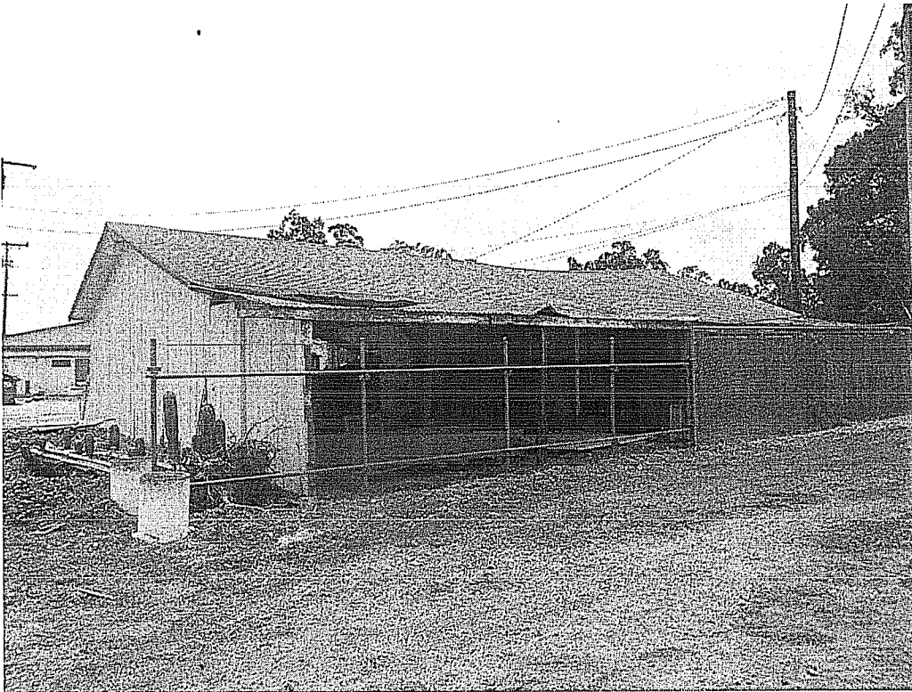
Figure 19 Shed/Equipment (looking east and north elevations)
