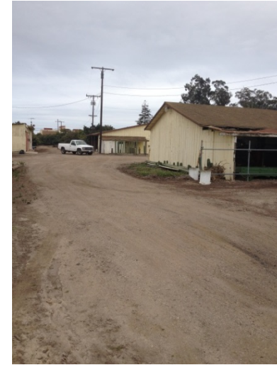
Photograph 9. View of the storage/workshop structure, facing south.
