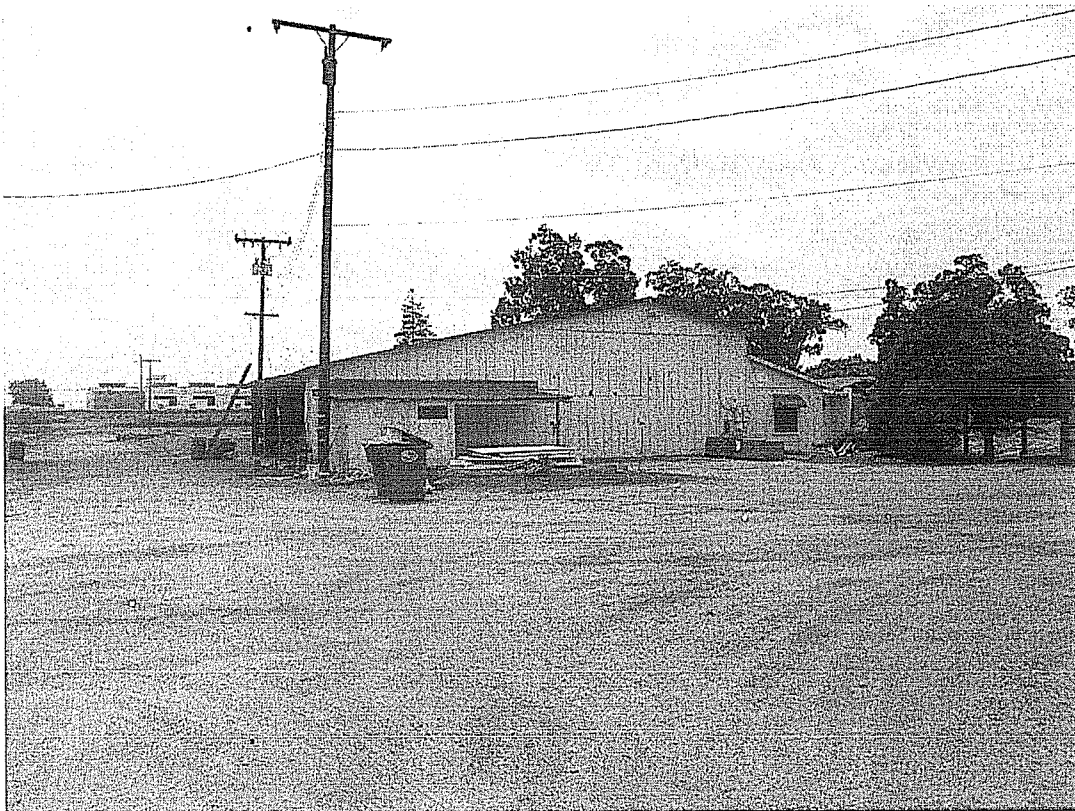
Figure 21 Shed/Equipment building, north elevation (looking south)
