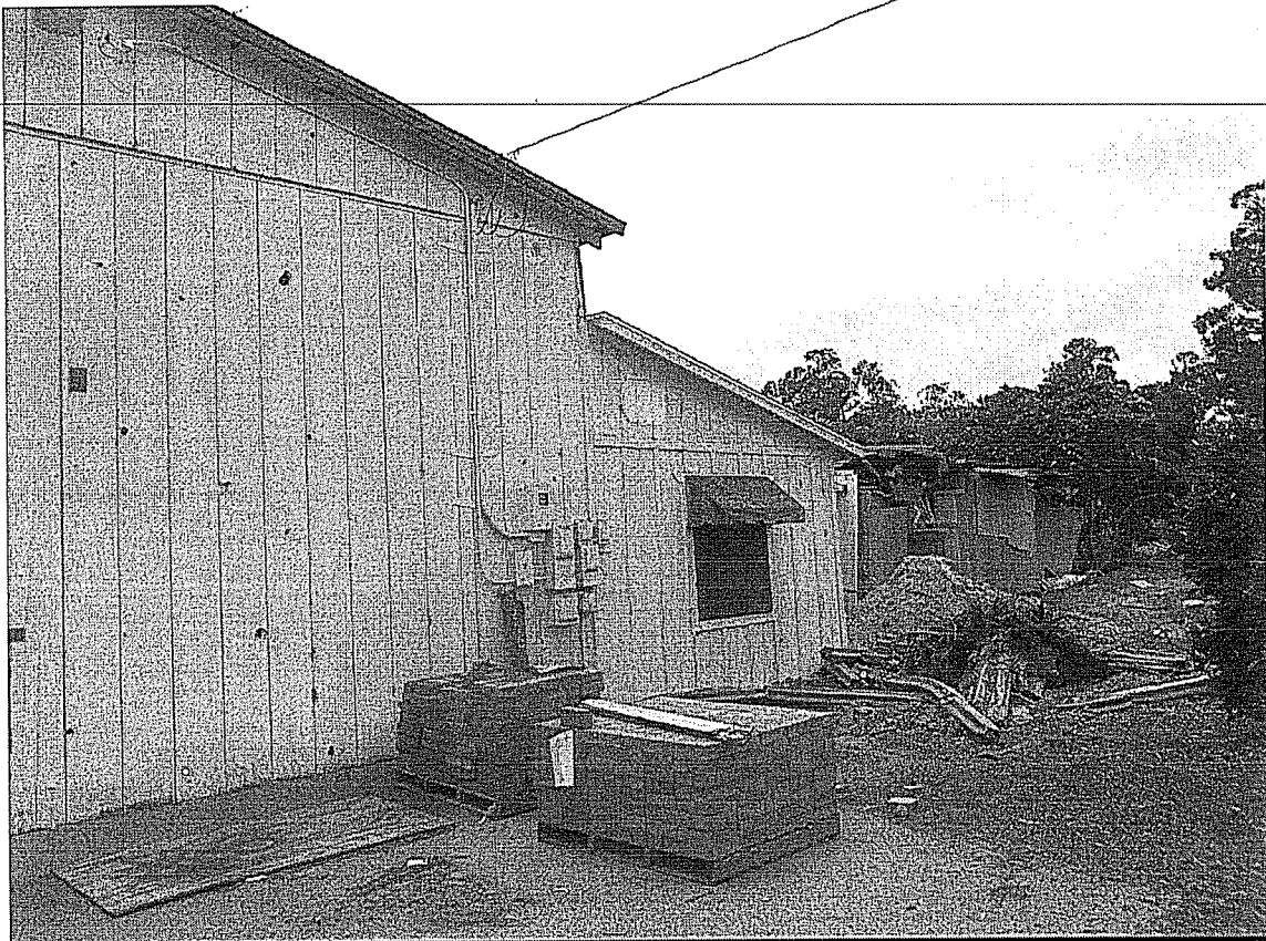
Figure 22 Barn/Living Quarters, west end of north elevation (looking southwest)
