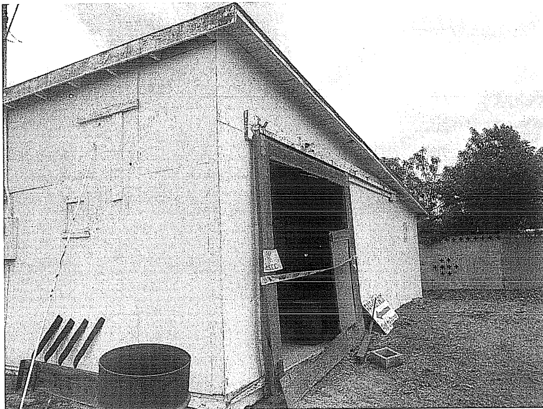
Figure 25 Shop/Equipment Storage Building, south elevation (looking east)
