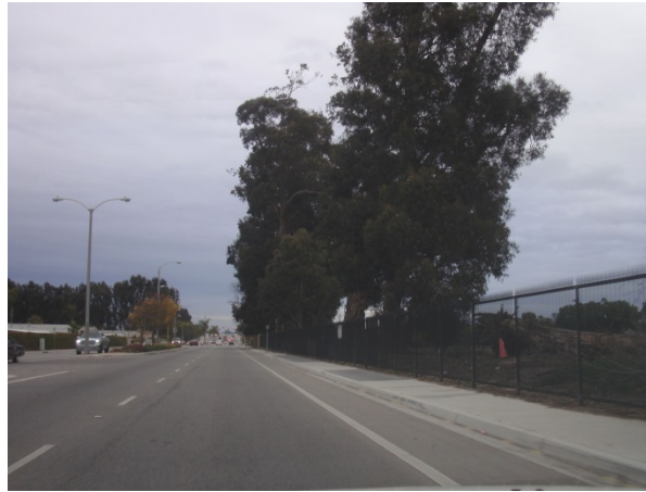
Photograph 14. View of the northern adjacent properties and E. Pleasant Valley Rd., facing northeast.
