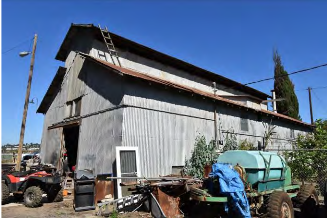
Barn No. 2, East and South Elevations
