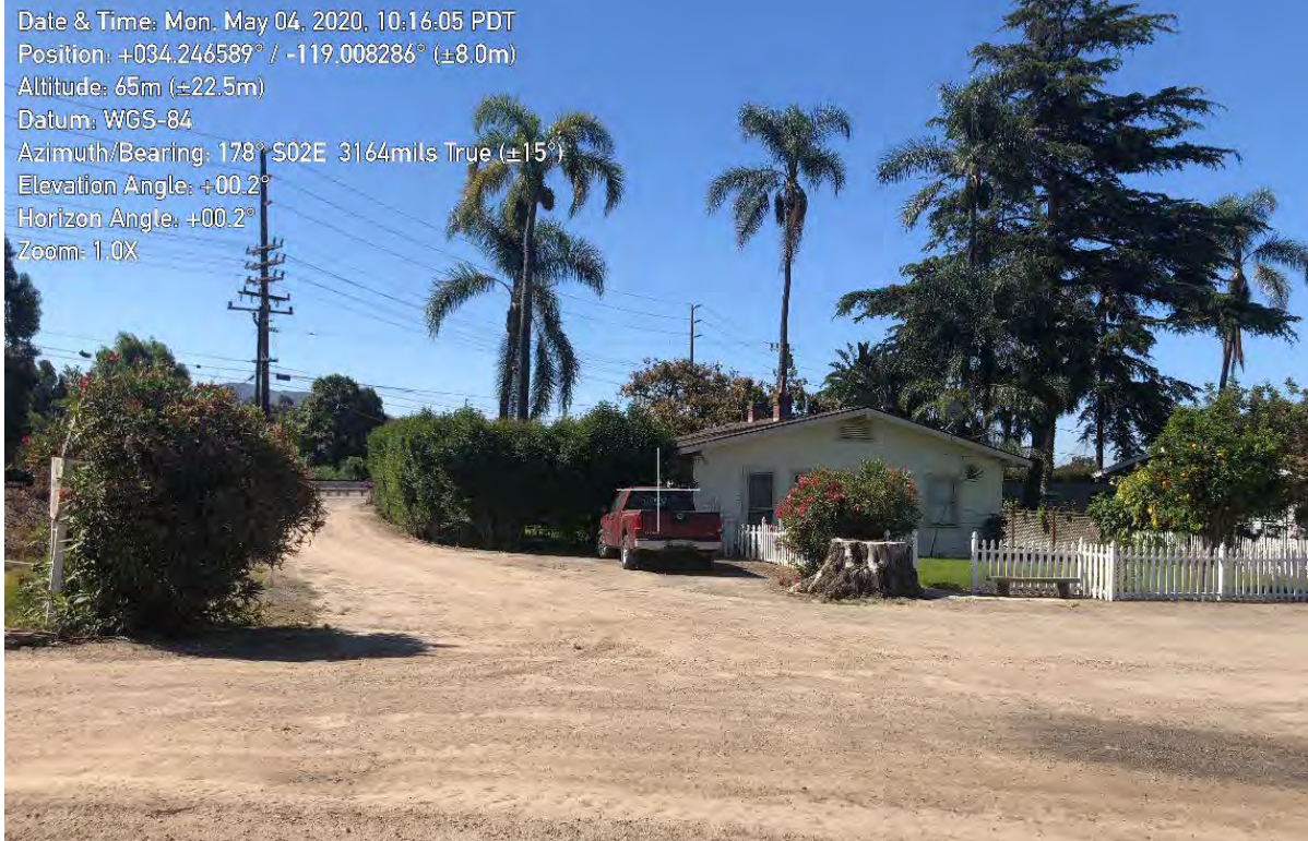
Photograph 9. (Photo point 6) View to south showing existing unpaved roads, structures, and ornamental vegetation.
