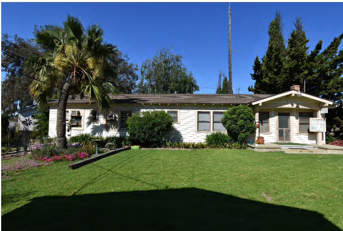
Figure 9 Residence No. 4, Primary (East) Elevation
