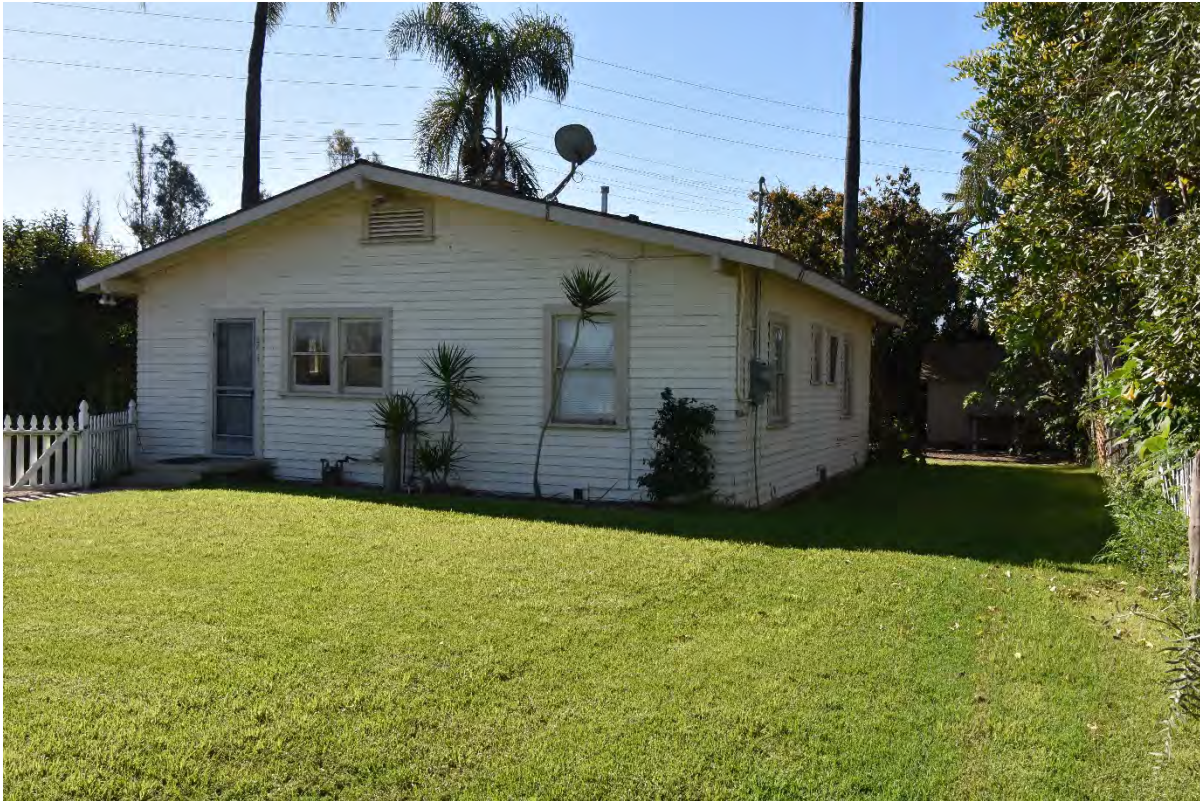
Figure 6 Residence No. 1, Primary (North) and West Elevations
