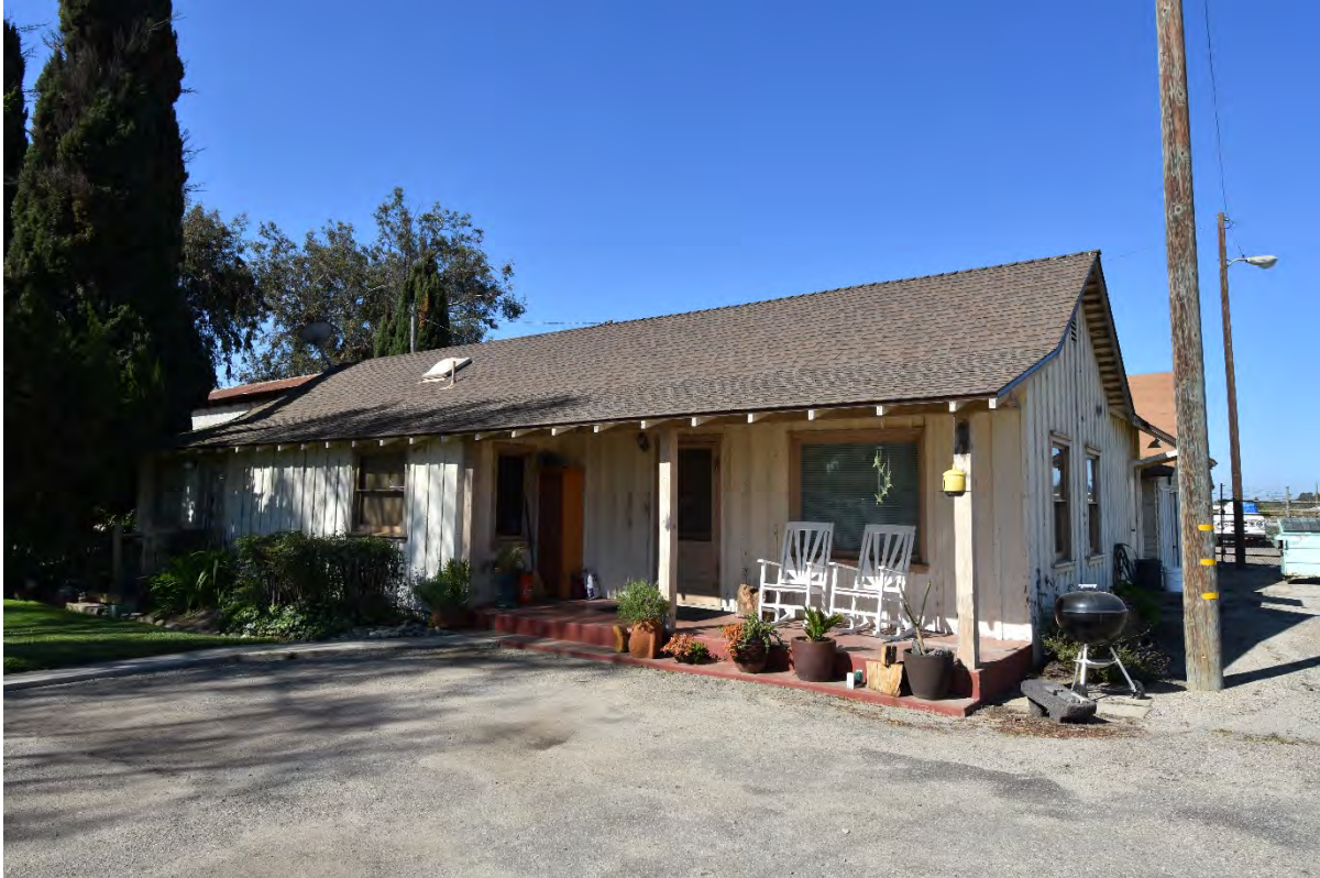
Figure 10 Residence No. 5, Primary (East) Elevation
