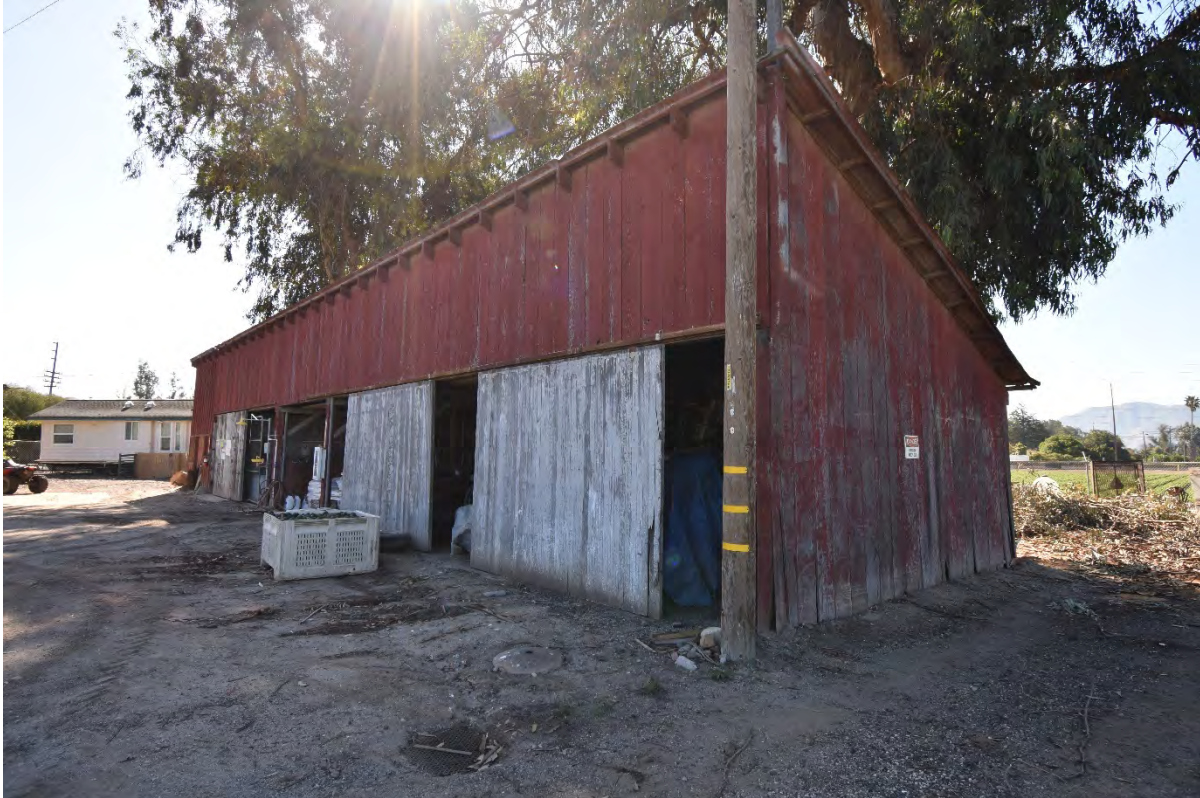
Figure 13 Barn No. 3, Primary (North) and West Elevations
