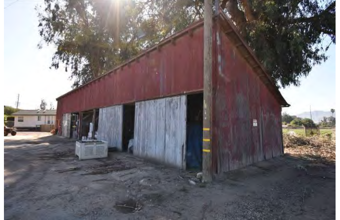
Barn No. 3, Primary (North) and West Elevations
