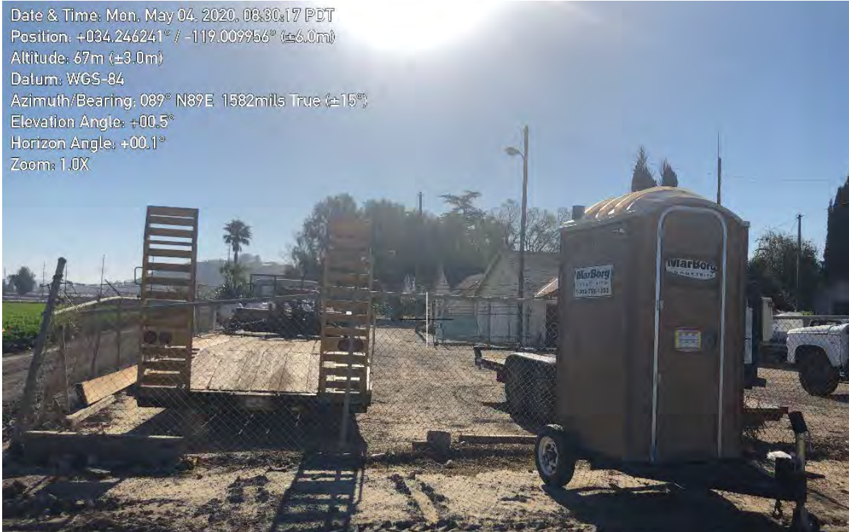
Photograph 1. (Photo point 1) View to east showing existing structures and unpaved parking area.
