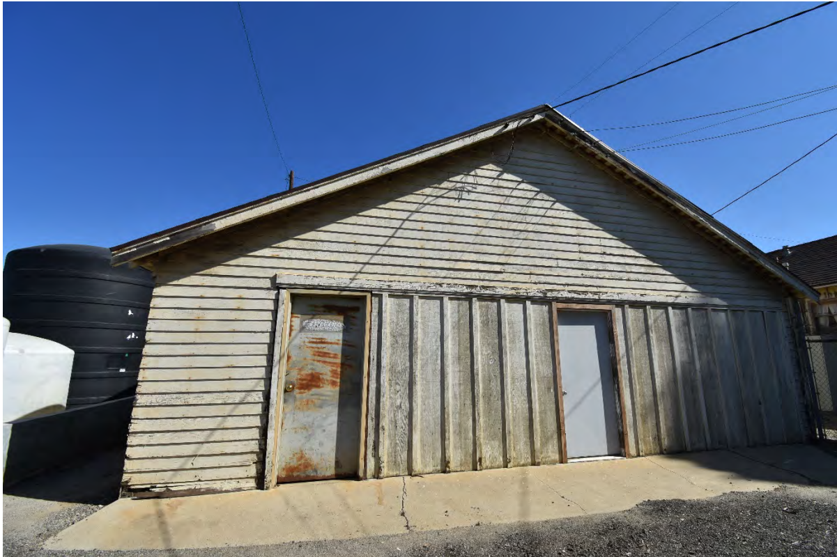
Figure 11 Barn No. 1, South Elevation
